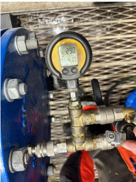
Photo 2. The pipe was pressurized with water up to 29 barg
